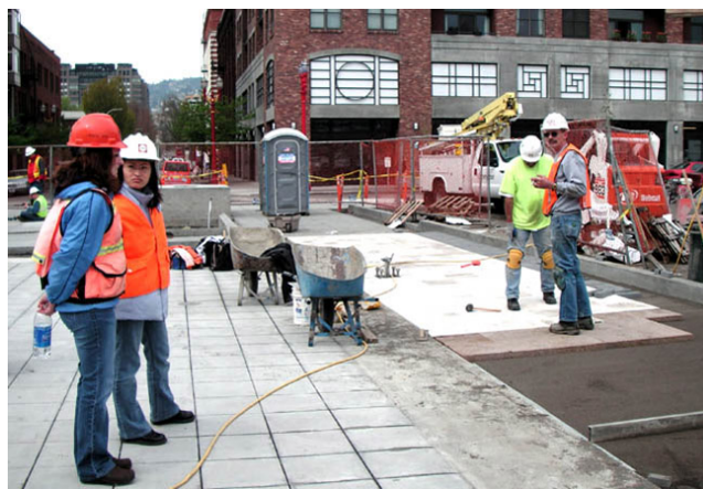
Figure 4 – Installing the sandset festival walkway pavers
