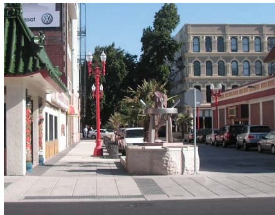
Figure 10 – Detectable warning panels across the sidewalk and on the wide curb ramp
