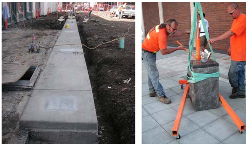
Figure 8 – Bollard beam with base plates (l); installation of a bollard (r)
