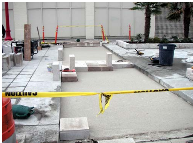
Figure 6 – Resetting the festival traffic pavers
